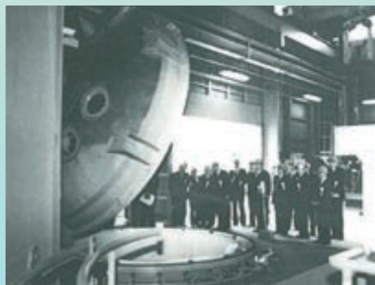
Rocket propellant production equipment completed in 1978 (Taketoyo Plant)
