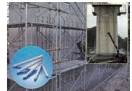
Example of use in an actual project (anti-earthquake reinforcement of Shinkansen bridge piers)
