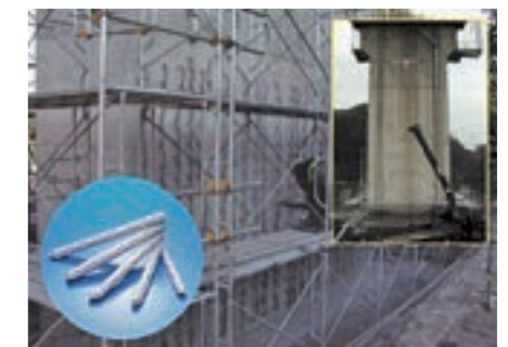
Example of use in an actual project (anti-earthquake reinforcement of Shinkansen bridge piers)
