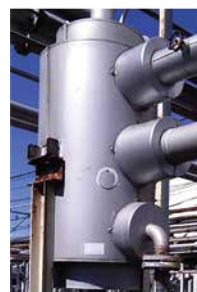
Condenser for PFC cooling and recovery (photo shows one attached to a PFC tank)
