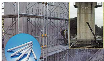
Example of installation (Shinkansen bridge piers anti-earthquake reinforcement work)
