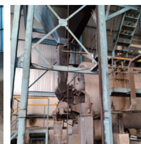
Boiler using biomass fuel
