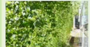
Participation in the Kawasaki City Green Office Promotion Council Creation of rooftop greenery, green walls, and greenery on our grounds
