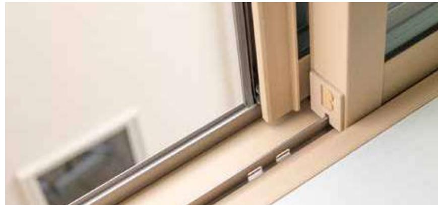
Window sashes made using vinyl chloride resin contribute to the spread of energy-efficient housing because of their excellent heat insulation. Organic peroxides are used as polymerization initiators for the vinyl chloride resin, and thus contribute to the spread of energy conservation.
