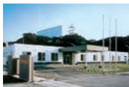
Tanegashima Plant on Tanegashima Island (Japan Aerospace Exploration Agency)
