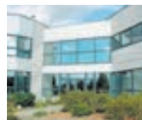
NOF METAL COATINGS EUROPE S.A. Head Office (in France)
